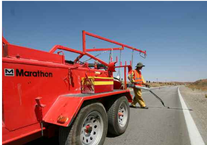
Burlington, Ontario-based Marathon Equipment puts its asphalt crack sealing machine to work in Shiraz, Iran.
